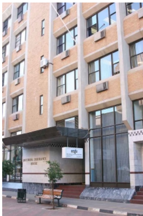
BOTA office building in Gaborone
