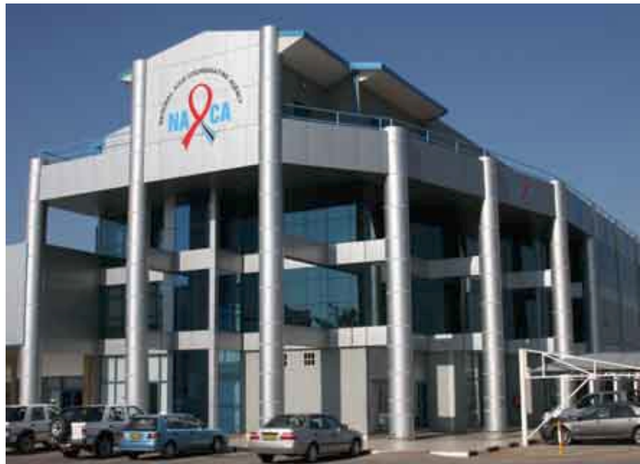
NACA office building in Gaborone
